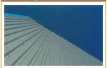
CA Groups SolarWall® is an astonishingly simple, effective solution to the demand for CO<sub>2</sub> reduction - and the energy cost savings that accompany it. A steel or aluminium cladding for industrial and commercial buildings that captures warmth from the sun and uses solar heated air to heat the building.
