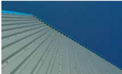
CA Groups SolarWall® is an astonishingly simple, effective solution to the demand for CO<sub>2</sub> reduction - and the energy cost savings that accompany it. A steel or aluminium cladding for industrial and commercial buildings that captures warmth from the sun and uses solar heated air to heat the building.
